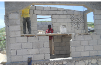
Almost done! One of the first PID houses built in Canaan nears completion.
