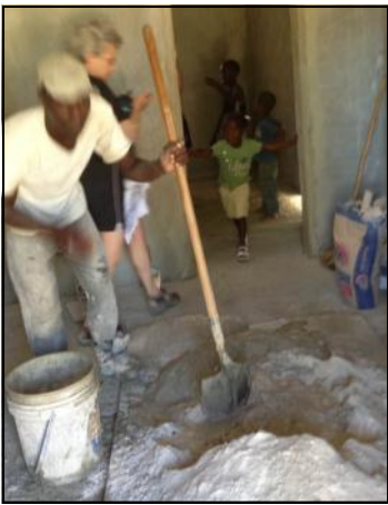
Putting the finishing touches on the house.
