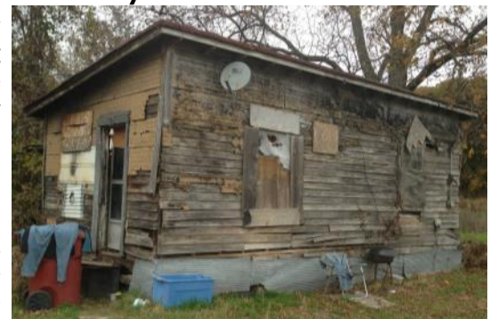
Glendora, Mississippi home in need of repair
